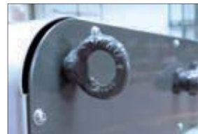
Detalle anclajes. View of fixtures.
