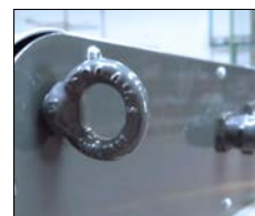
Detalle anclajes. View of fixtures.
